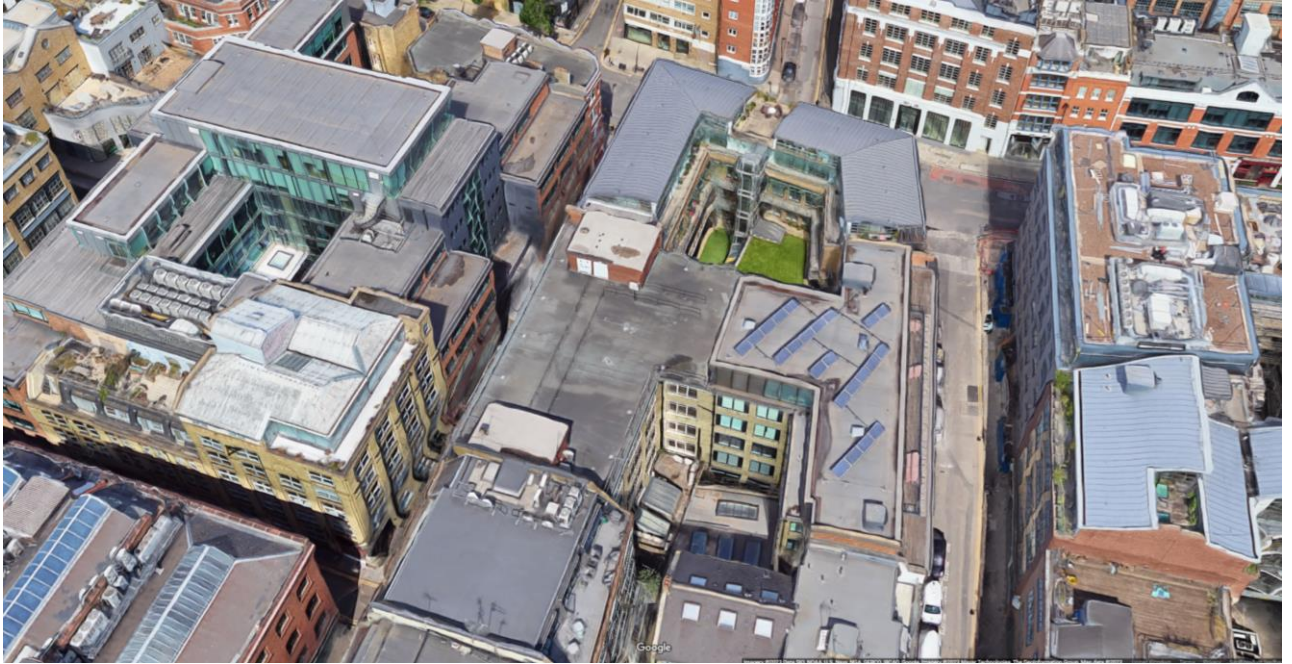
Figure 4: view of internal courtyards.
